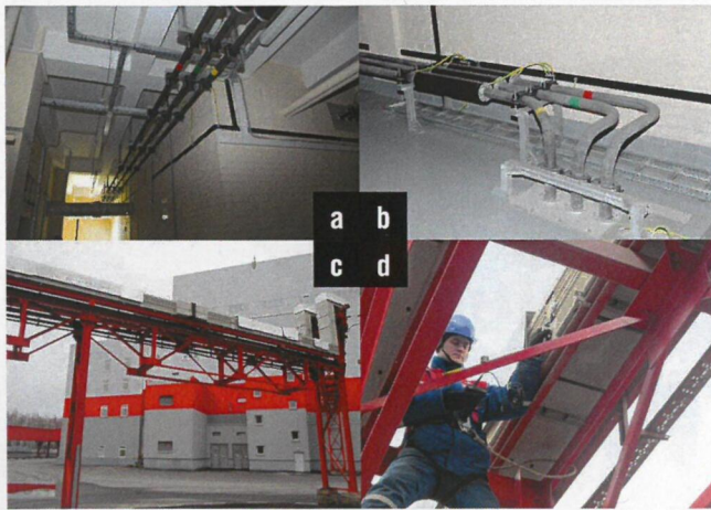
Fig.3 — Current conductors with cast insulation 6 kV: a), b) — PICRIB type; c), d) — CRIB type
